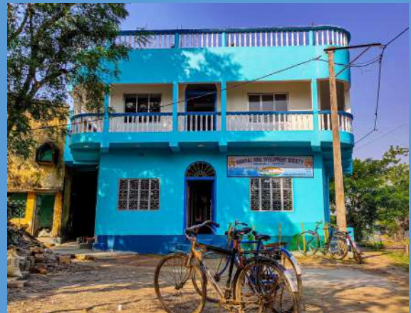
New Panikhali School building completed
